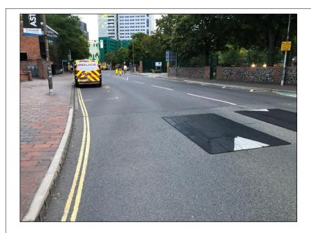
A new cycle lane is detailed around the Police parking bay directly adjacent to the speed cushions. Vehicles will not be able to straddle the speed cushion at an angle to avoid the cycle lane resulting in conflict with cyclists in the lane. The Police parking bay should be relocated, and the scheme amended to remove the conflict.
