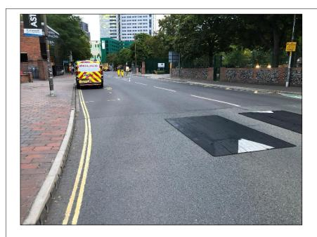
A new cycle lane with satellite island is detailed similar to the opposite side of the road. There is only 2.5m carriageway width adjacent to the speed cushion to accommodate the cycle lane and island (3.2m wide on opposite side of road). This reduced width will result in an inadequate width cycle lane and insufficient clearance adjacent to the existing speed cushion for cycles and vehicles to pass safely. Amend design to suit available carriageway width.
